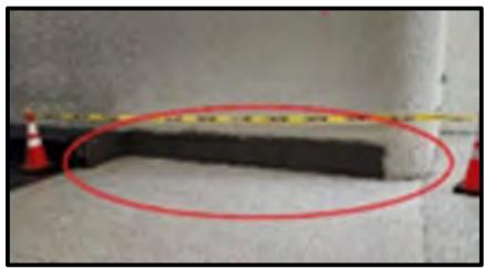
This project entailed the cutting, squaring and patching of a stationary tiled bench outside Door No. 12. Additional work entailed ensuring the bench was flushed and sprayed to blend in with the existing wall. The repair improves vision and contributes to a safer environment. The task was completed on January 27, 2025.
